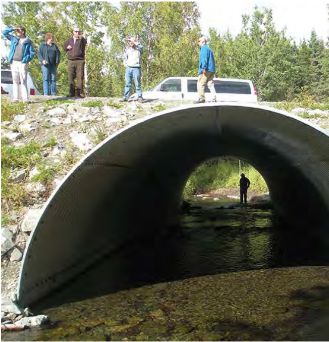
Photograph 4-3: Completed Open Bottom Steel Arch Culvert
