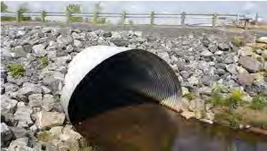
Photograph 4-5: Typical Steel Arch Culvert
