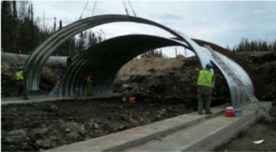
Photograph 4-2: Open Bottom Steel Arch Culvert Under Construction
