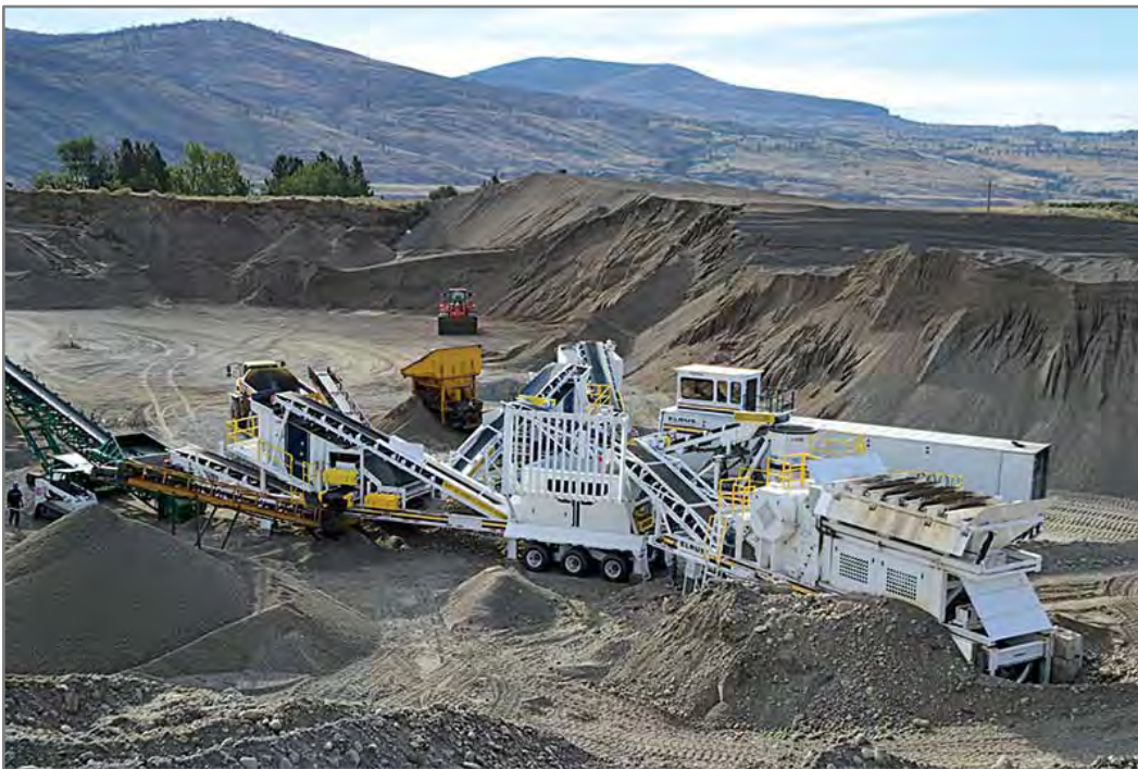
Photograph 4-7: Typical Potable Crushing Plant
